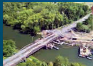
UK: Nuneham rail viaduct restoration, Network Rail.
