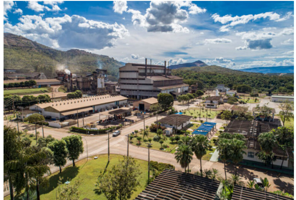
Aerial view of the Codemin ferronickel operation and surrounding area in Niquelândia, Brazil.
