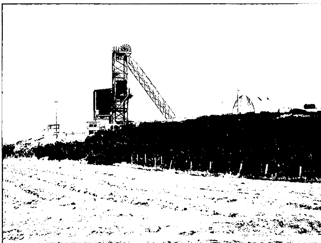
Parys Mountain headframe and winder house
