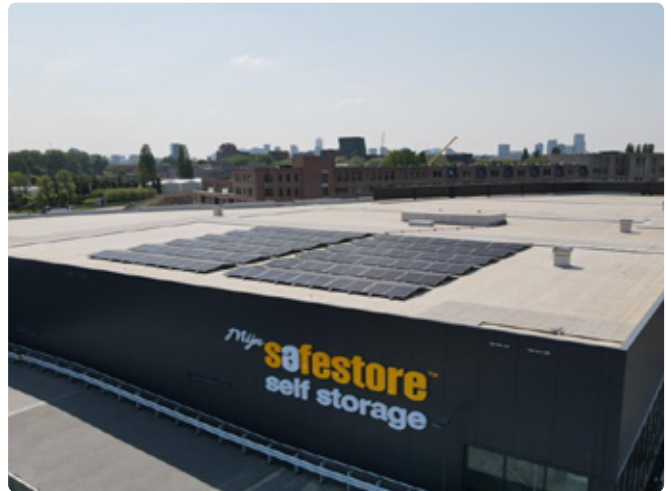
Rotterdam with a new PV Cell system.
