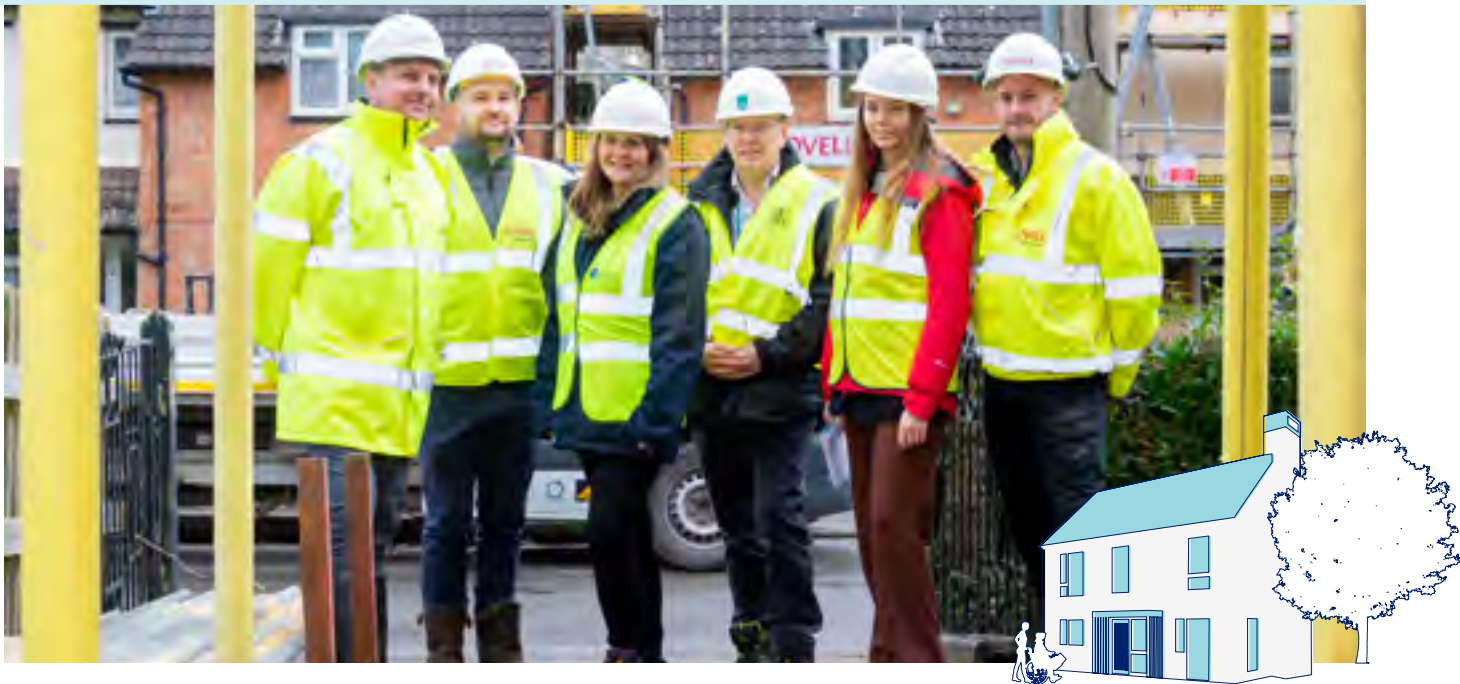
Jeanette Hodges, Head of of Carbon and Operations, with representatives from the Department of Business, Energy, and Industrial Strategy (BEIS) visiting the retrofitting works in Henley-in-Arden, Warwickshire
