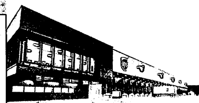
A state-of-the-art and highly automated 450,000 sq ft warehouse let to UPS (Image courtesy of McLaughlin & Harvey developer)
