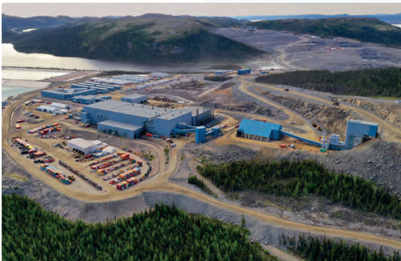
Vale - Voisey's Bay mine
