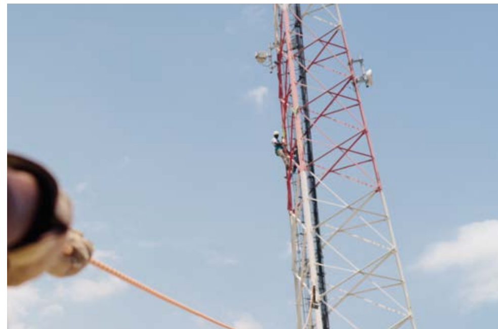
Lifting equipment up a tower using a mechanical hoist.
