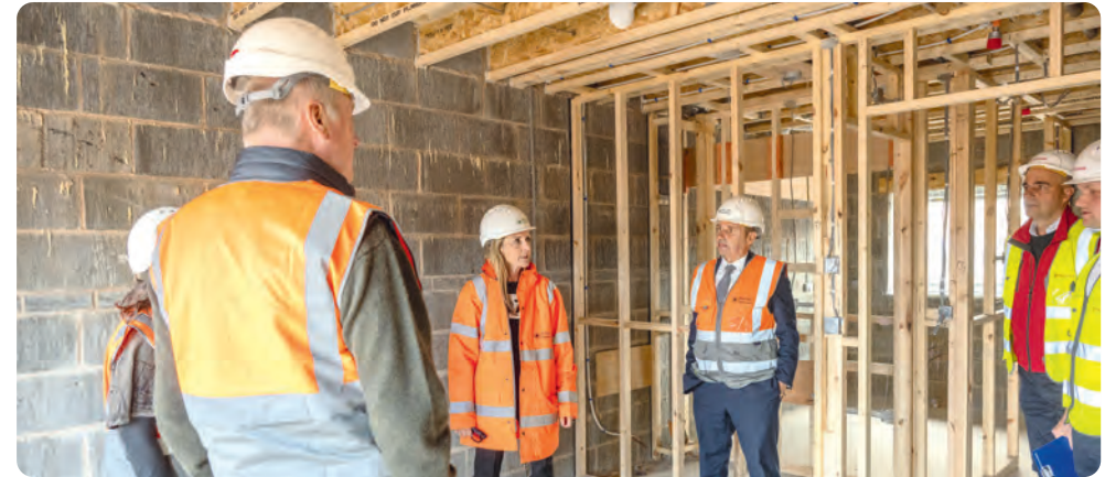
Board members visiting one of our developments to review health, safety and environmental performance, inspect ongoing structural works, and observe how safety and quality standards are being maintained throughout the delivery of the remaining phases
