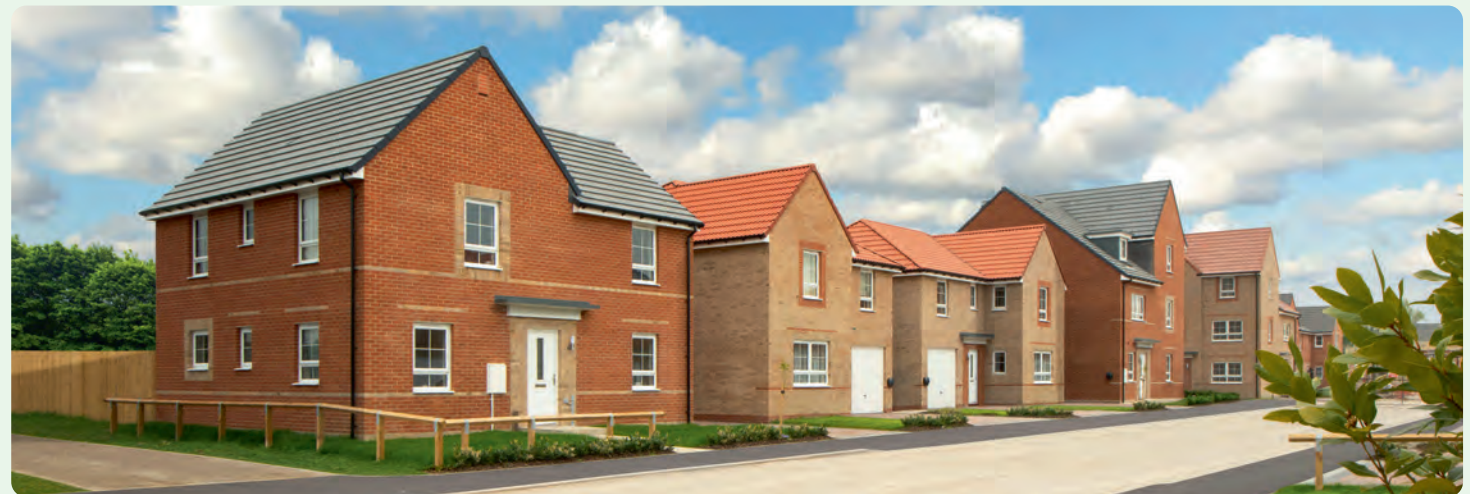
Barratt Homes at Stewart's Reach, Pocklington, Yorkshire
