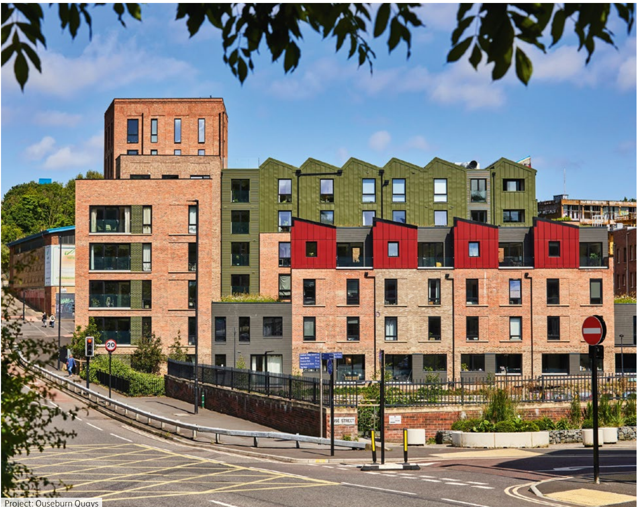
Project: Ouseburn Quays
